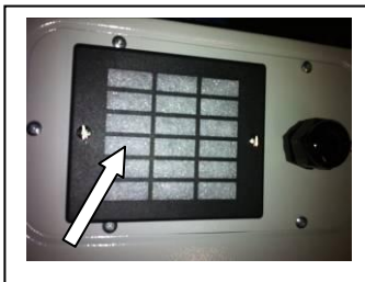
Fig 1 - Electric Panel Filter
