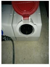
WALL SOCKET 3 PHASE MAINS **SUPPLY** NEEDS TO BE 5 PIN 32AMP **OUTLET**
